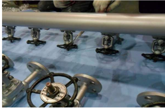
steam manifold with valves
