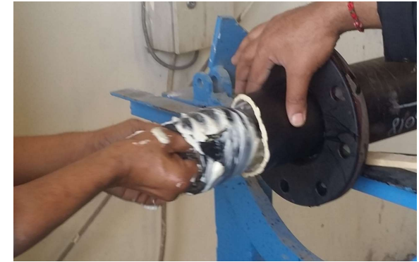
fixing a rubber lining tube to a small pipe
