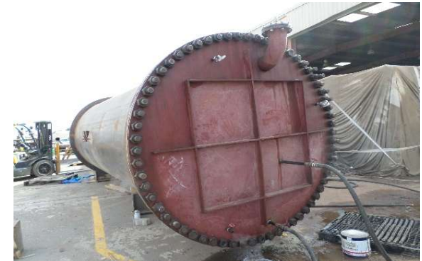
open curing of rubber lined pipes
